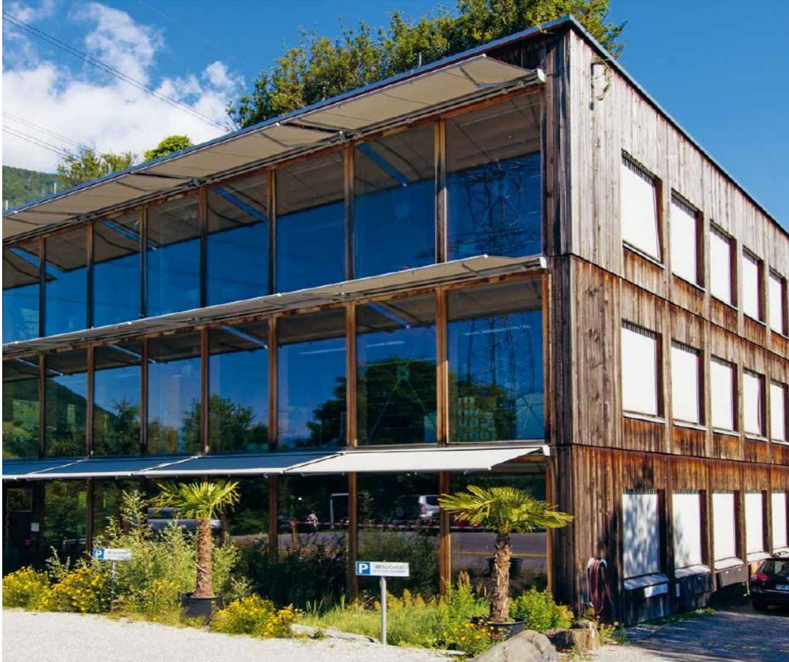
Figure 1: External shading protection from heat in the summer (EIV, 2018, p. 82)
